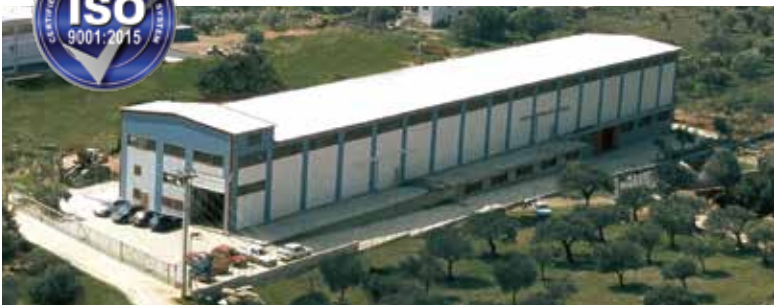
SAFEDOOR FACTORY AT KALIVIA, ATTICA
