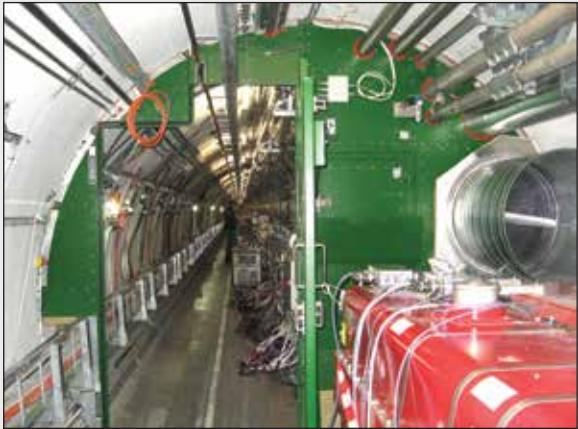
Specialized fire barriers for the CERN tunnel
